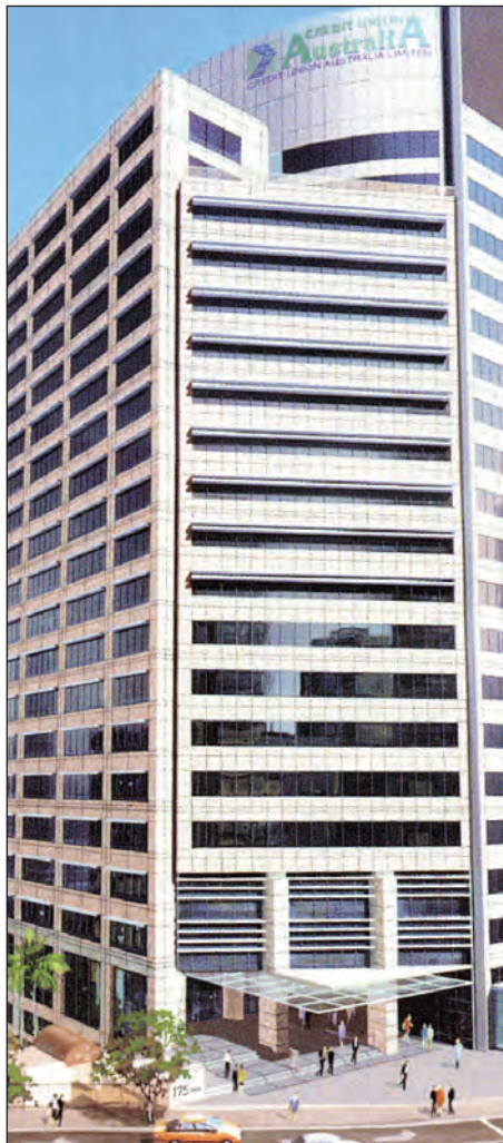
175 Eagle Street – Australia's first thinking building – on which Hutchies set a new building record.
